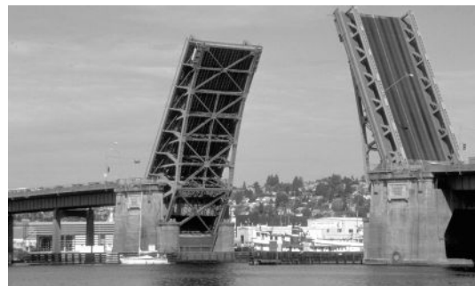
A bascule bridge opening for shipping
