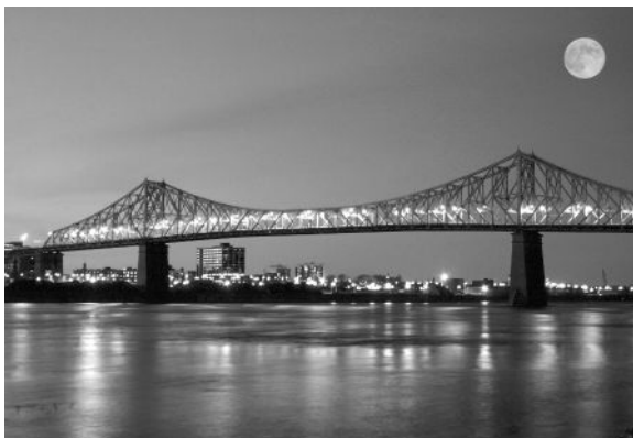
Jacques-Cartier Bridge, Montreal, Canada: a cantilever bridge that incorporates a supporting steel truss structure.
