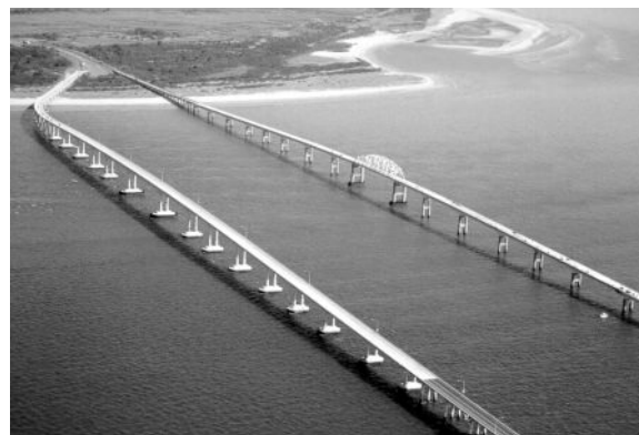
Photo Courtesy of the Chesapeake Bay Bridge-Tunnel
